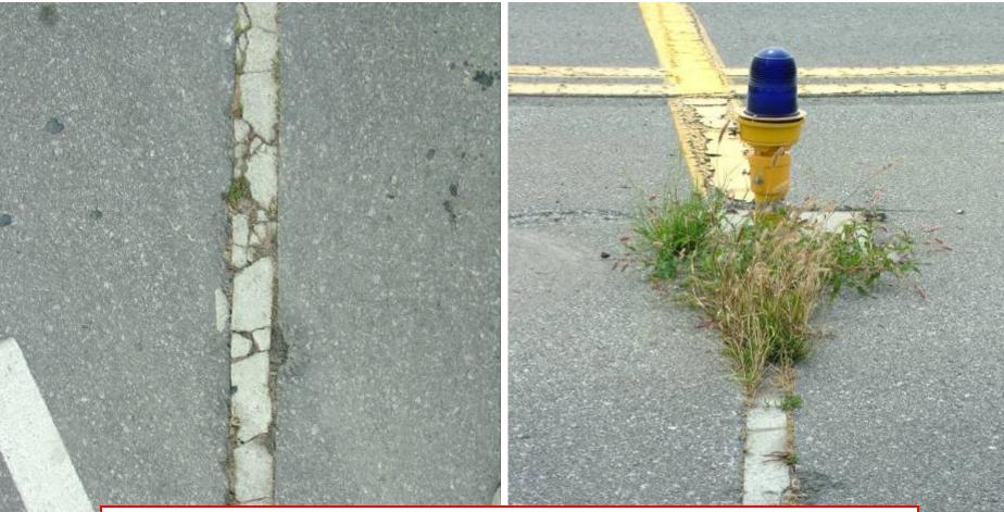
Pavement failure along trenches as a result of inadequate backfill material (Rapid set mortar, which solidifies in one week to provide full strength).
