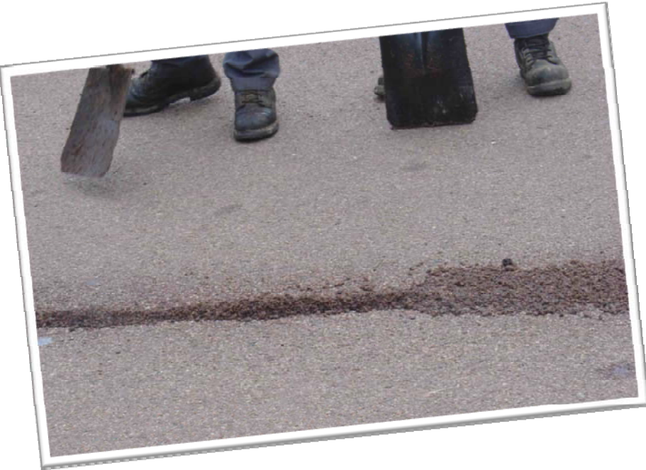
Heated fresh material is added to the heated deteriorated joint
