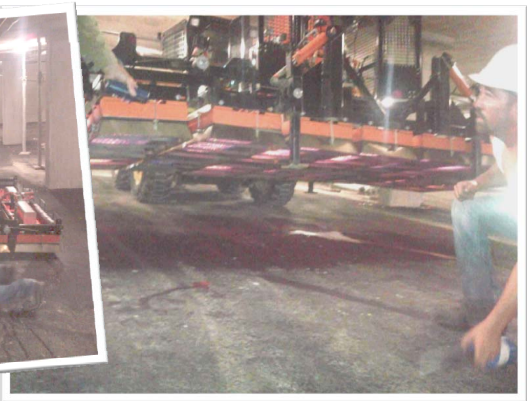
Check asphalt temperature with infrared gun
